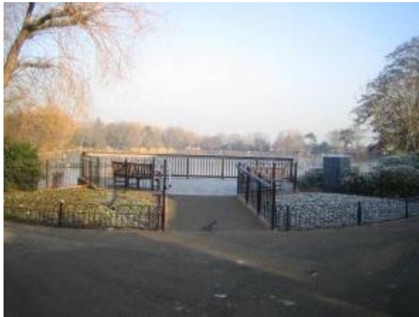
Viewing platform installed in 2006
