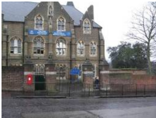
The original entrance with brick piers and stone coping
