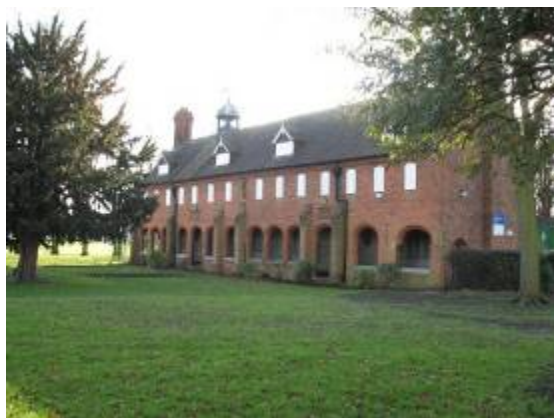
View of the Chapel buildings
