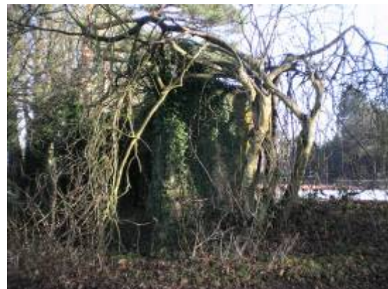
The fig and remains of the kitchen garden wall by the tennis courts
